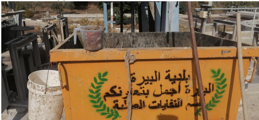
Photo (2): container of screen 20 mm in Al Bireh WWTP
